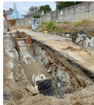
Travaux Naval Group - Lanester
